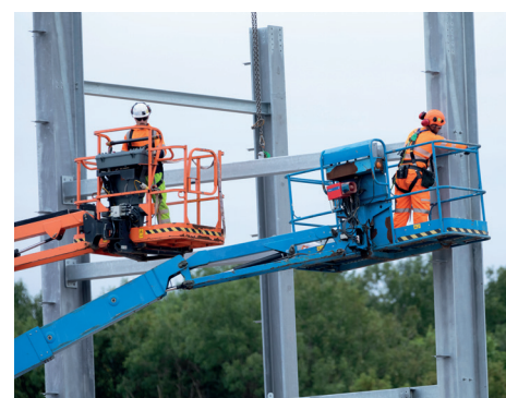
Workers erecting the framework of one of Sofia's converter station buildings
