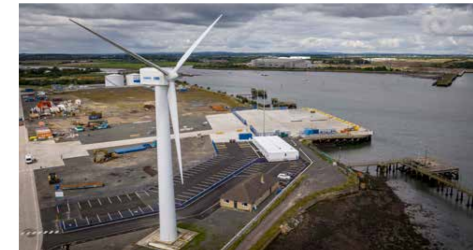
Bates Clean Energy Terminal, Port of Blyth (Photo: Mike Smith)
