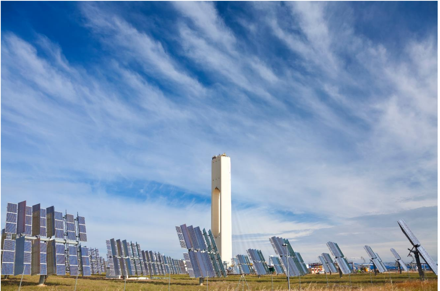
Massive solar array at Seville in S. Spain – Europe's first commercial solar power plant of its type
